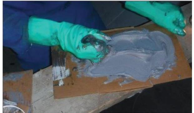
*Devcon Titanium Putty resin & hardener mixed on board for filling & fairing defects*
