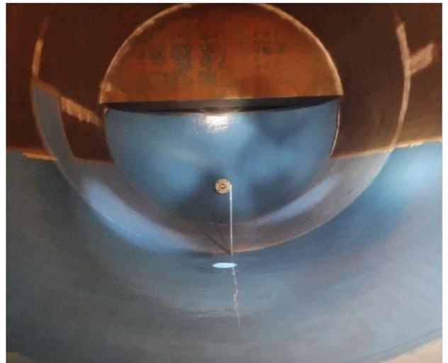
*Restored vessel interior after application of Devcon Titanium Putty & Devcon Brushable Ceramic Blue*
