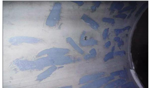
*Devcon Titanium Putty applied over damaged areas inside pressure vessel*
